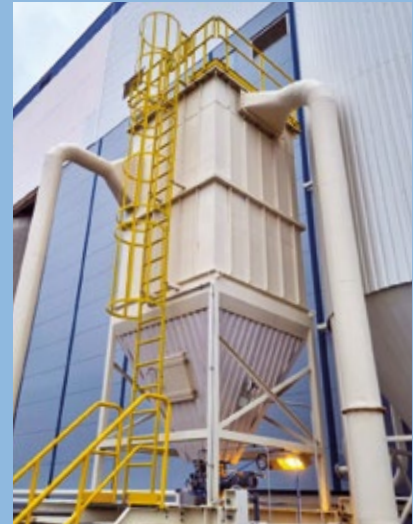
Photo: Example dust filter at Sotkamo plant.
